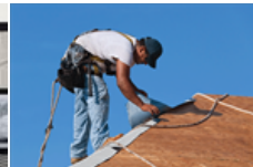
Fall Protection: Residential Roofers an OSHA Priority
