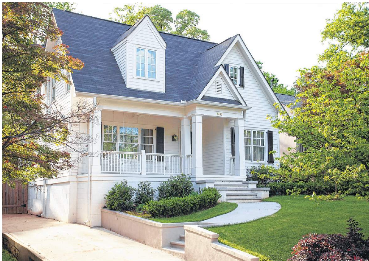
A new second story on a Loring Heights home in Atlanta features a dormer and revised roof pitch, updating the former one-story home. CONTRIBUTED BY GLAZER CONSTRUCTION
